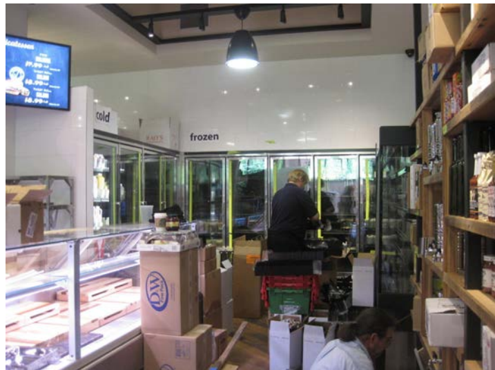
Market area under construction.
